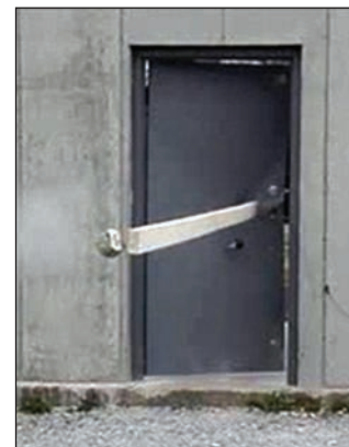
Tornado safe room impact test results: Door assembly failed at latch/lock
